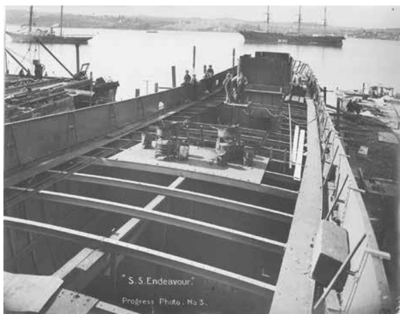
Figure 3. Construction of FIS Endeavour at Cockatoo Island Dockyard, August 1908 [Photo: CSIRO Archives]
