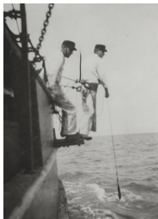
Figure 5. The execution of a (manual) sounding, in this case on board HNLMS Ever (source: NIMH)
